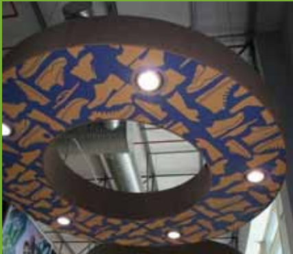
Ceiling Bulkheads and Lighting
